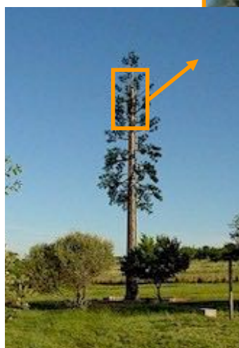
Hiding the the BSE pylon by means of a "giant" artificial tree
