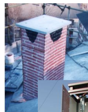
BSE hidden within a chimneypot-like cover for over-the building applications
